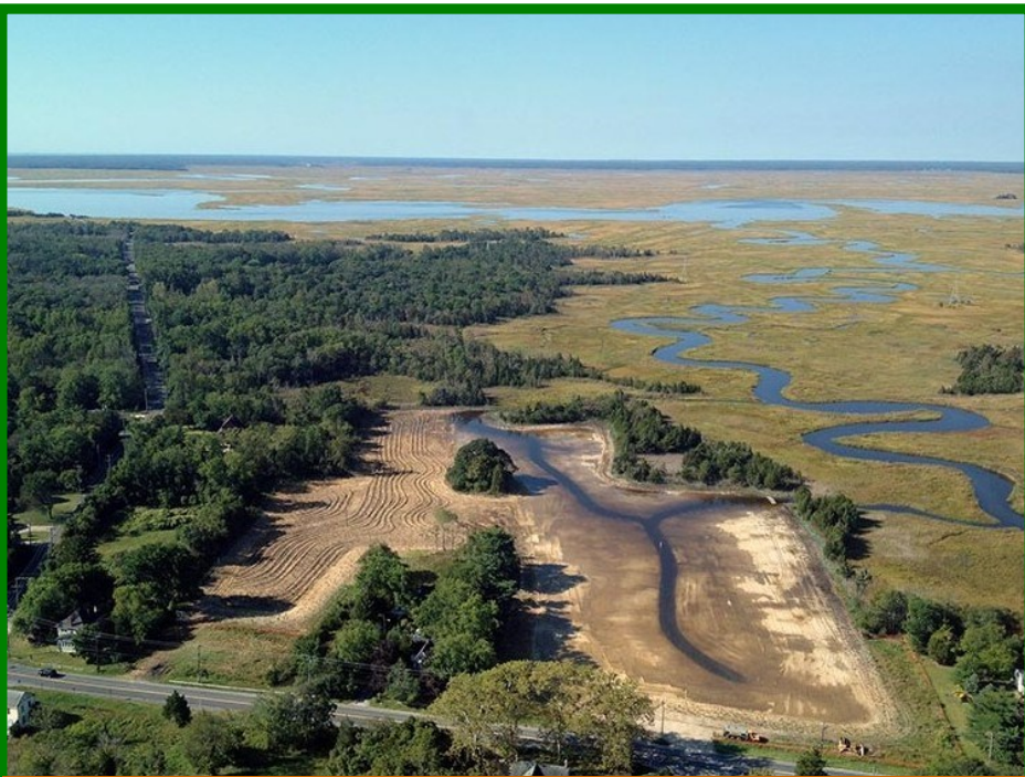
May 30, 2013 Aerial view looking southwest over the Lakes Creek Wetland Mitigation Bank site. The topsoil is being stripped and materials are being loaded for transport to the county stockpile site.
