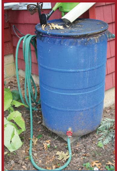
**One of Three 55 Gallon Rain Barrels Capturing Runoff from the Roof of My House**
