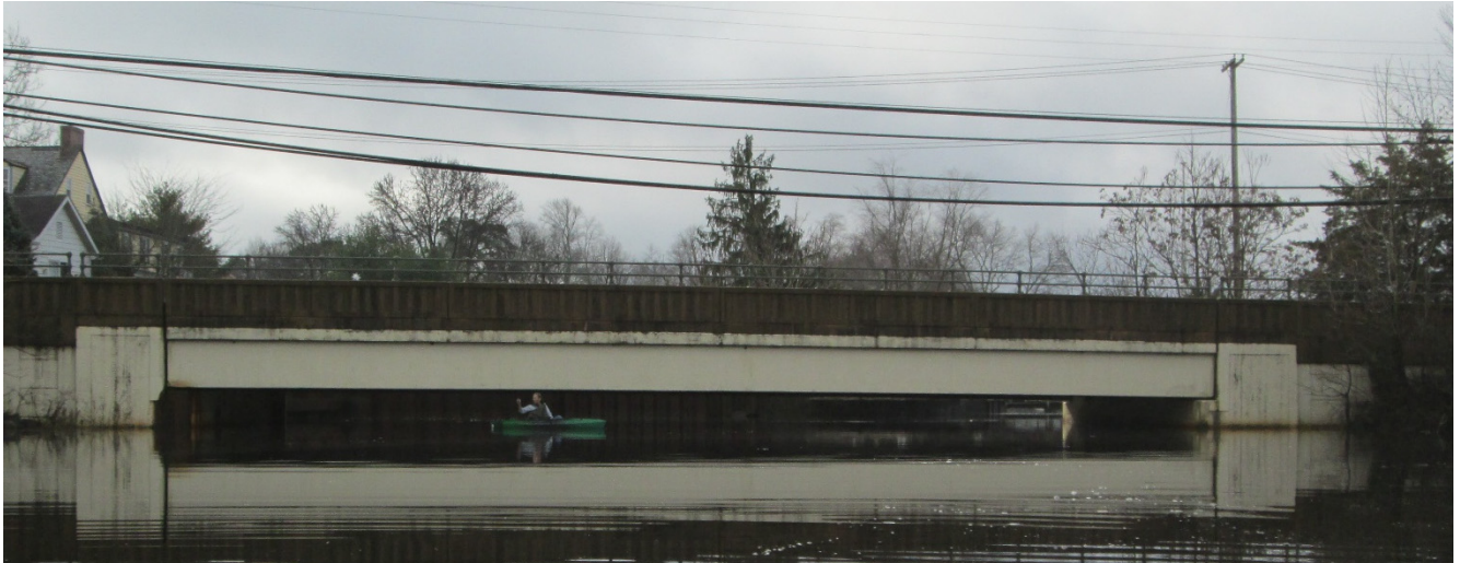
P1: 12/25/15, 12:19 pm, upstream view of State Route 40 bridge in Mays Landing with 186 square feet of unobstructed area.
