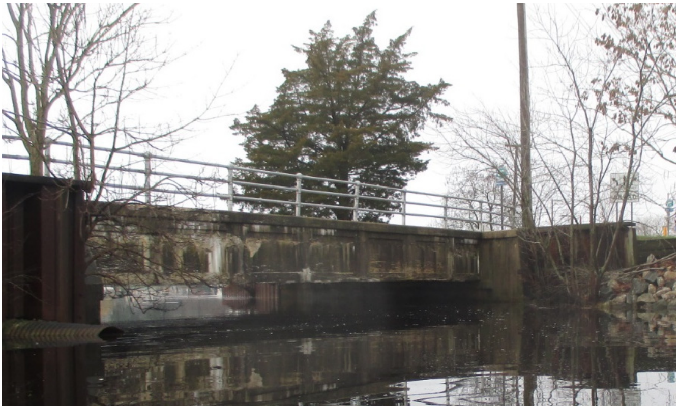
P2: 12/25/15, 12:04 pm, upstream view of County Route 559 bridge in Mays Landing with 96 square feet of unobstructed area.
