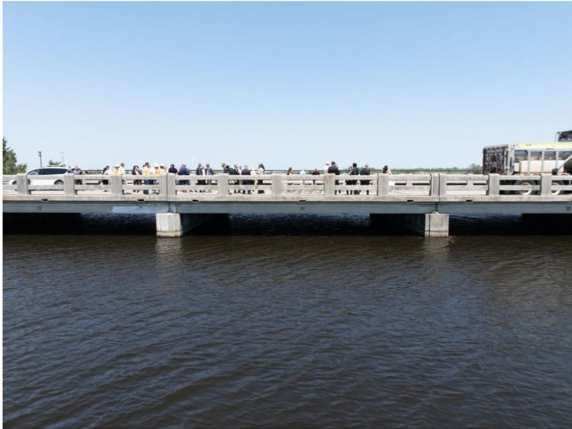
Aerial view of Cedar Swamp Creek Bridge on route 50, a location set for a NJDOT replacement project, which is the first project being built under the innovative Design-Build project delivery method, seen here after a press conference on May 20, 2026.
